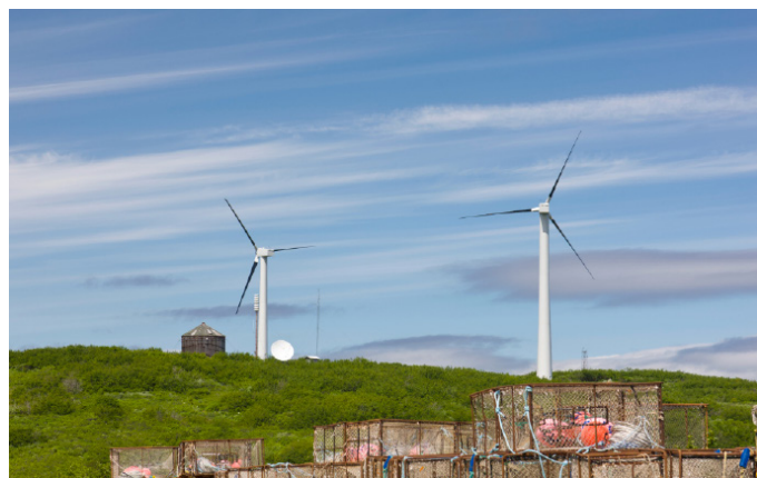
Vestas V39 turbines, photo courtesy of Rich Stromberg, AEA.
