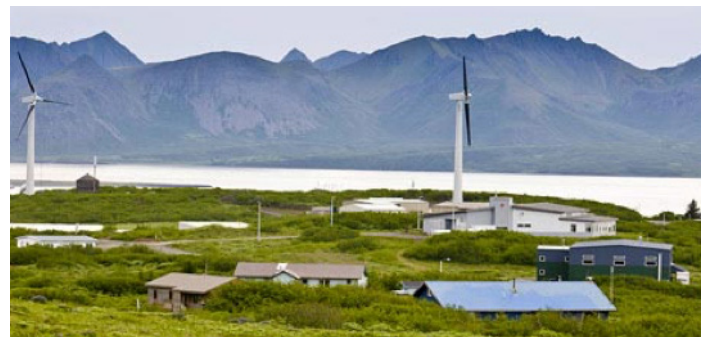
Vestas V39 turbines, photo courtesy of Rich Stromberg, AEA.
